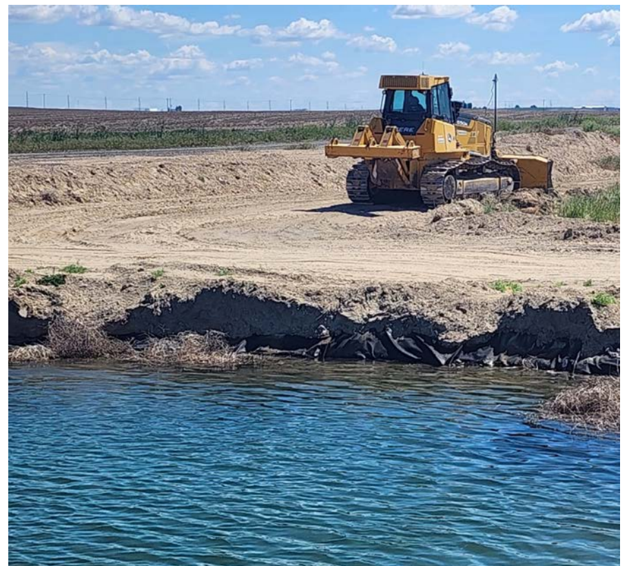
The end of the canal prior to EL 86.4.
