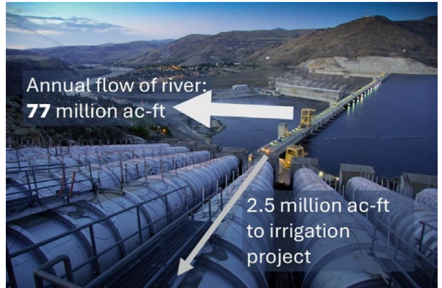
Figure 4. The pumping station at Grand Coulee Dam, which supplies water to the Columbia Basin Irrigation Project. The amount delivered to the project annually, 2.4 million acre-ft, is just 3% of the annual flow of the river at this location. Photo credit: United States Bureau of Reclamation.
