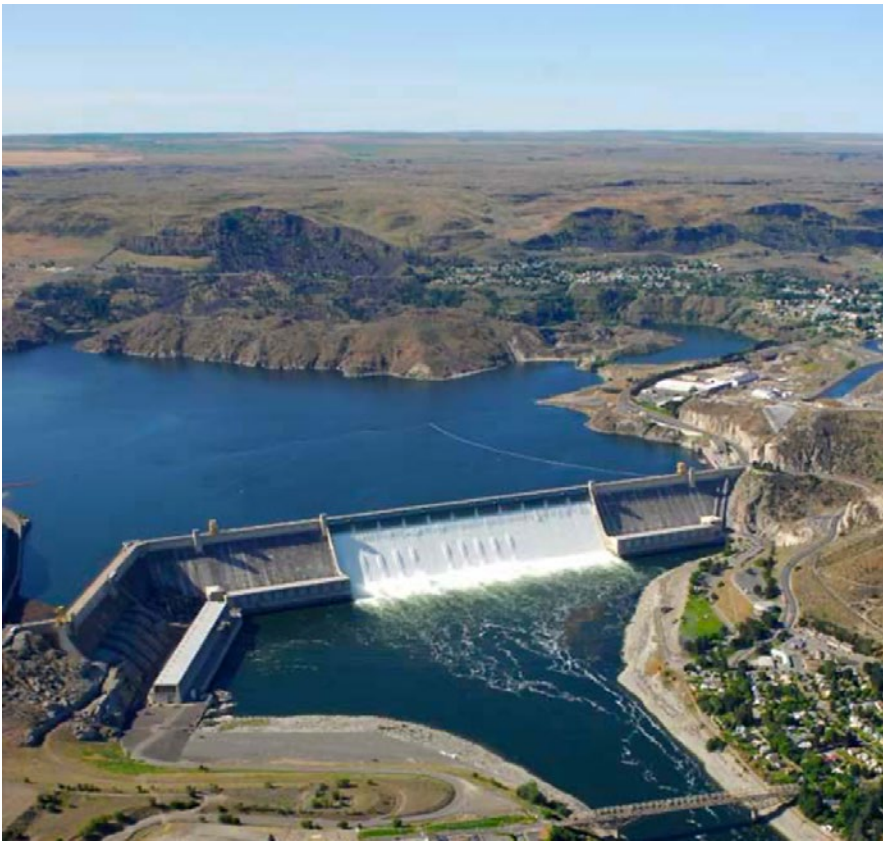
Figure 3. Grand Coulee Dam. Although the dam was completed in 1942, water did not flow to the Columbia Basin irrigation project until 1952. The pumping plant that lifts water to a canal that begins the irrigation project is just to the right of the dam. Behind the dam, Lake Roosevelt backs up all the way to Canada, storing 9 million acre-ft of water. Photo Credit: United States Bureau of Reclamation.
